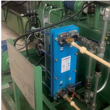
Oil Cooler in a Rolling Mill
