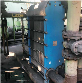
Condensate Heat Recovery in an Alumina Refinery
