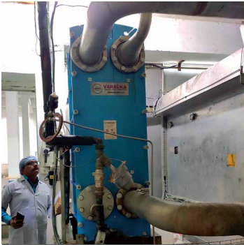
Steriliser PHE at API Pharmaceutical Plant
