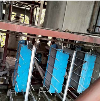
Formaldehyde Plant in a Wood Plywood Facility
