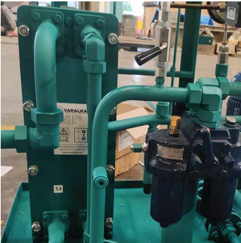
Gear Box Oil Cooling System
