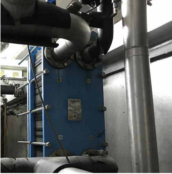
Hot Water PHEs at Pharmaceutical Plant
